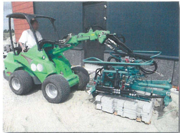
Paving flexible & cost efficient with a loader
