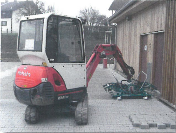
Highly competitive paving with 1.6 tonn machine
